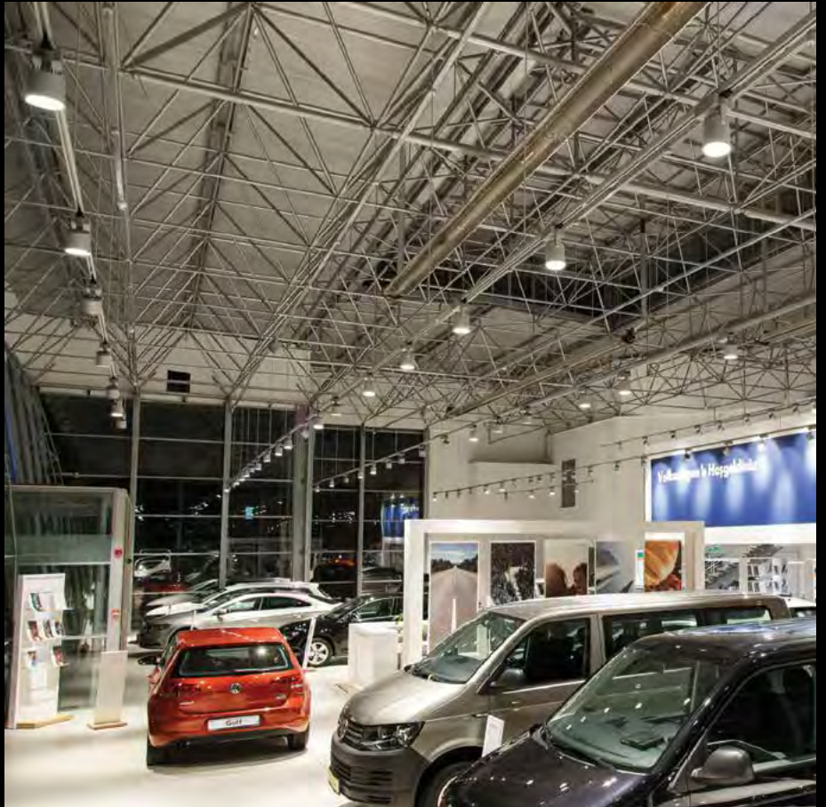
Lux level on the cars planned in average 1200lux.
