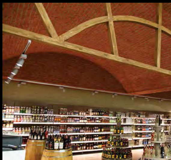
Single asymmetric LED lines provided excellent even light distribution on the wall whereas wide beam angle tracklights chosen to illuminate the beverage shelves.
